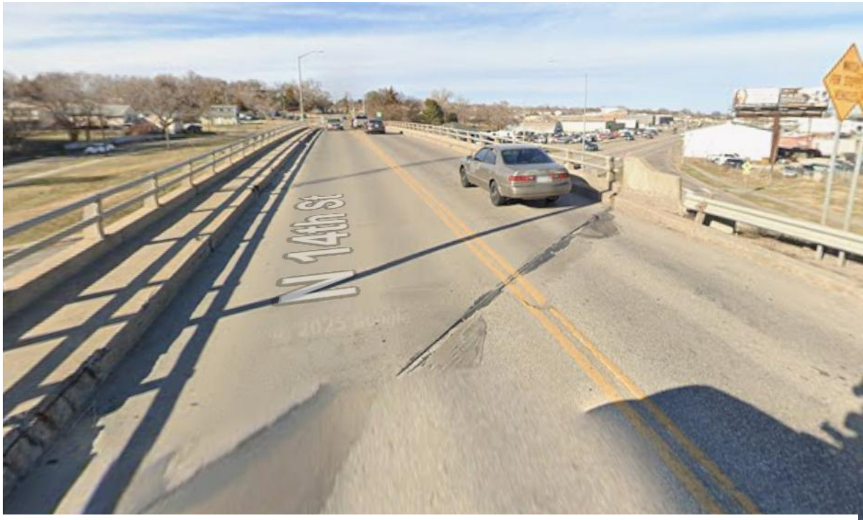
North 14 th Street Bridge looking north.
